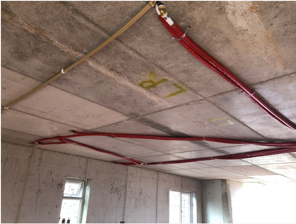
Photograph 5 – House numbers 1-4. Plumbing being installed. Internal fit out commencing.
