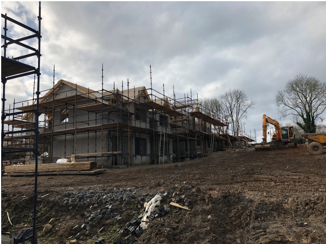
Photograph 2 – House numbers 9 – 16 incl. Roofing ongoing. Final phase of Sup-R-Wall being installed.
