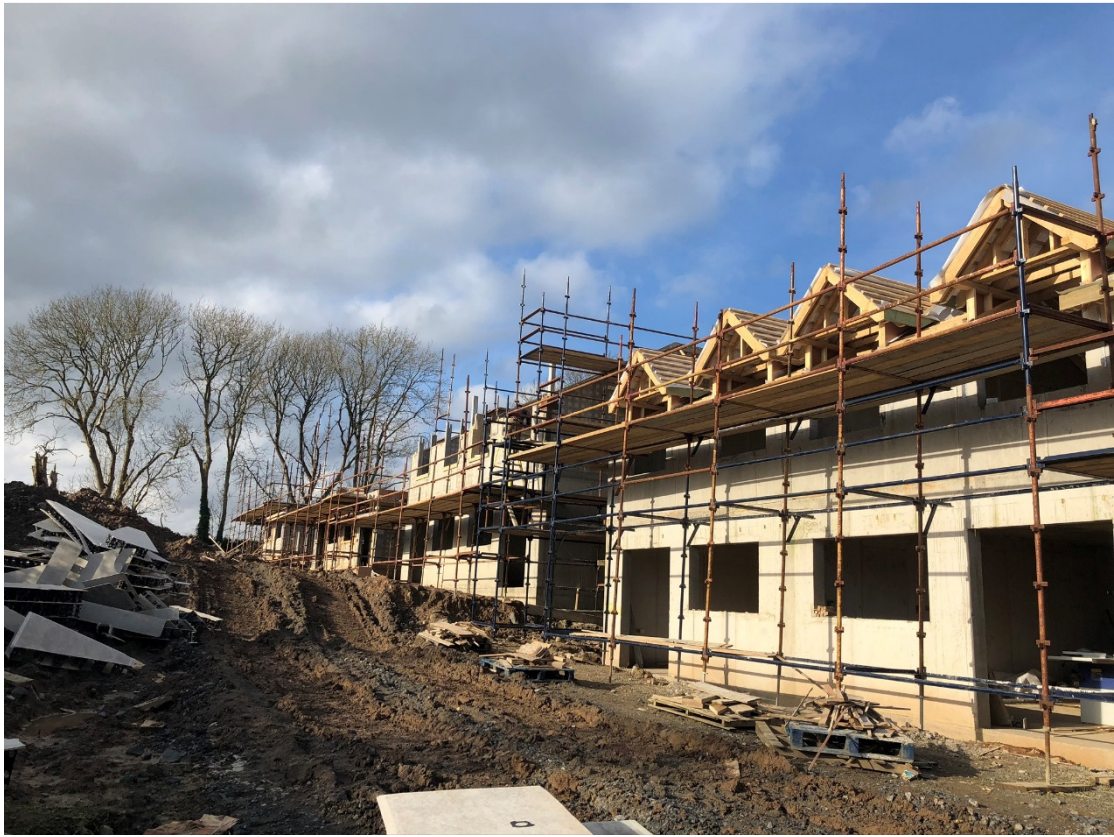
Photograph 3 – House numbers 9 – 16 incl. Roofing ongoing. Final phase of Sup-R-Wall being installed.
