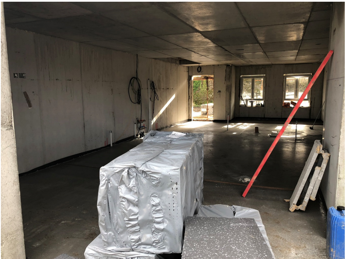
Photograph 4 – House numbers 1-4. Ground Floor & underfloor heating pipes installed.
